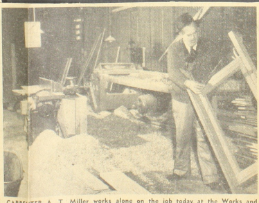
CARPENTER A. T. Miller works alone on the job today at the Works and Housing Depot, Salmon Street, Port Melbourne. Work at the store had been declared black because the Building Workers' Industrial Union says that Miller is unfranchised. Miller previously worked at Craig's Building. The job there was also declared black. Miller says: "My only crime is that I was forthright in my criticism of Communists."
